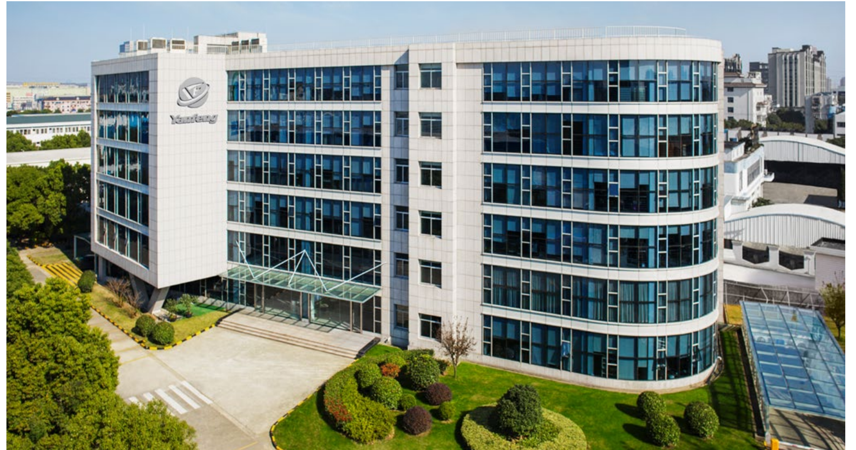
Our corporate headquarters in Shanghai, China.
